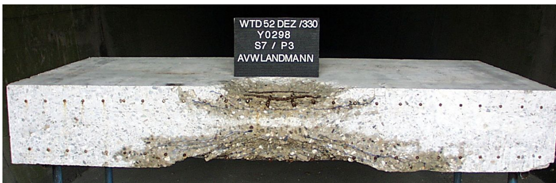
Figure 5: Cross section of damaged RC-slab (partly wet) [14]
