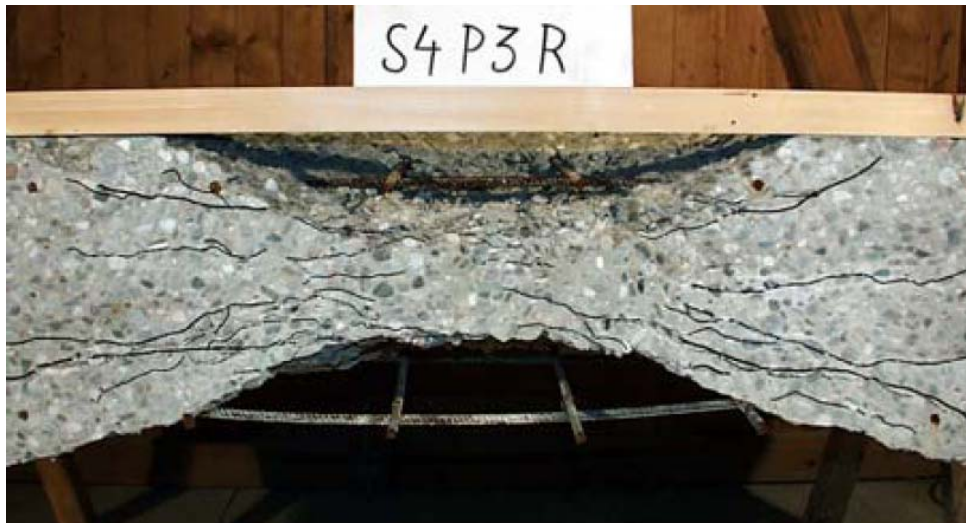
Figure 2: Damage after contact detonation [7]
