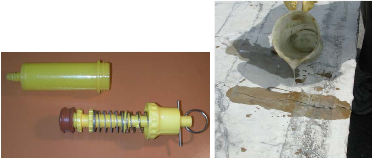
Figure 3: Injector for low pressure grouting (left) and repair by soaking (right)
